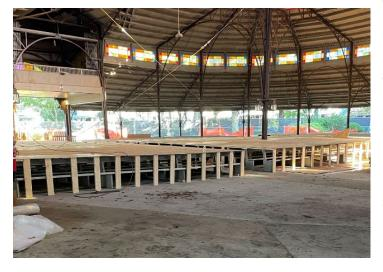
The Tabernacle benches are in the process of being protected in place for the duration of construction. A system of scaffolding is being built over the benches to ensure no damage occurs. This structure will be supported by dimensional lumber and have a layer of foam between the plywood covering and the bench seat backs. No portion of this protection structure is being secured into the benches themselves.
