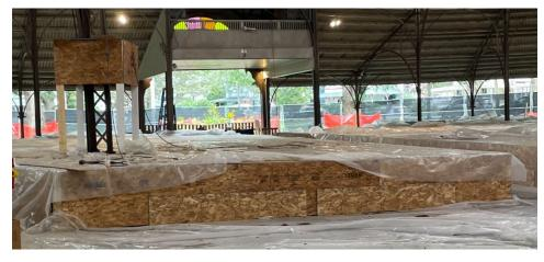
A box-like structure has been built around the glass lantern lighting fixtures to protect them. Plywood will also be secured over the stained-glass windows prior to work commencing in that area. Stage railings have already been protected.
